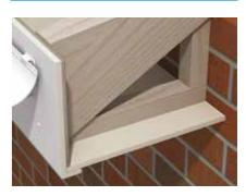
9mm capping board with 9mm utility board, fitted to a new 6mm plywood substrate
