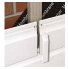
Butt joint trims can be used instead of joint trims providing they are staggered and fitted where a batten is located
