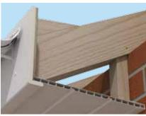
9mm capping board and 300mm hollow
